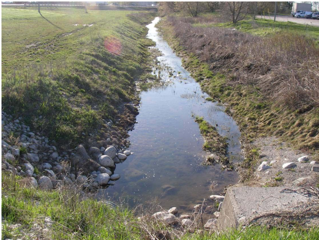
Photo 4. Apr 28, 2006 - View looking downstream from McKinlay driveway at trapezoidal channel. Note the wide nature of the channel and the early growth of bank vegetation which includes shrub plantings.
