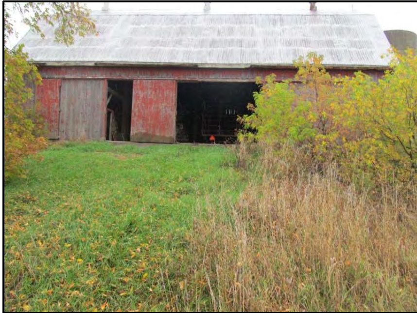
Photo 1 – View of Site Building A.
