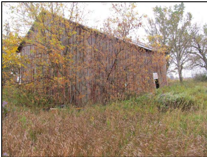
Photo 2 – View of Site Building B.
