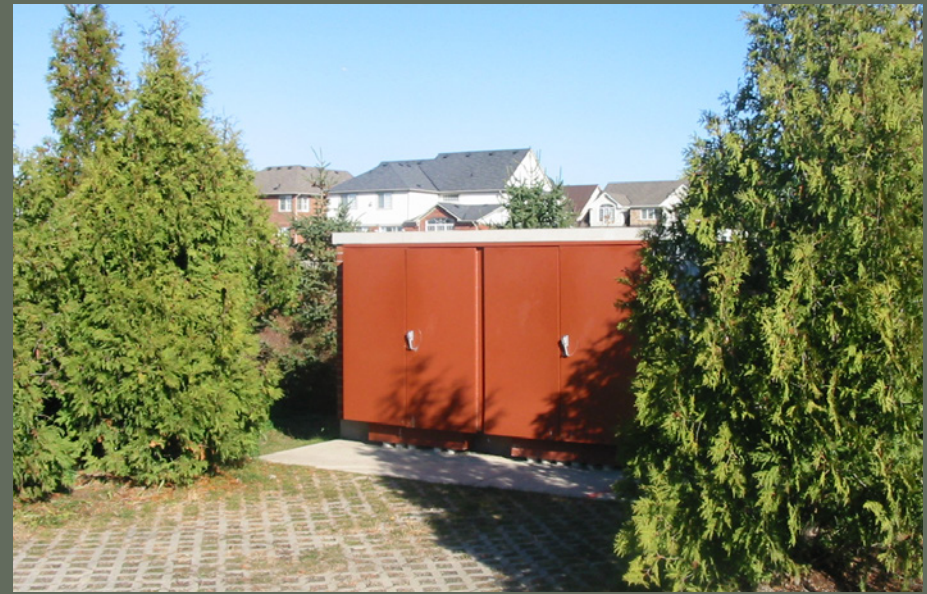
Image example of a Bell CUE unit partially screened within landscape features.
