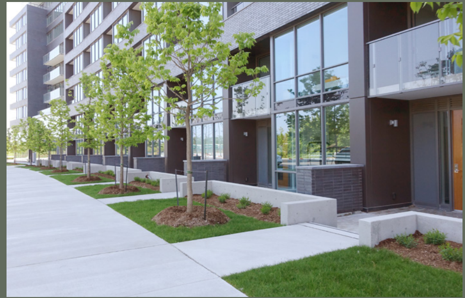
Image example of a individual walkway connections to ground condo apartment units, integrated with the architectural style of the building.
