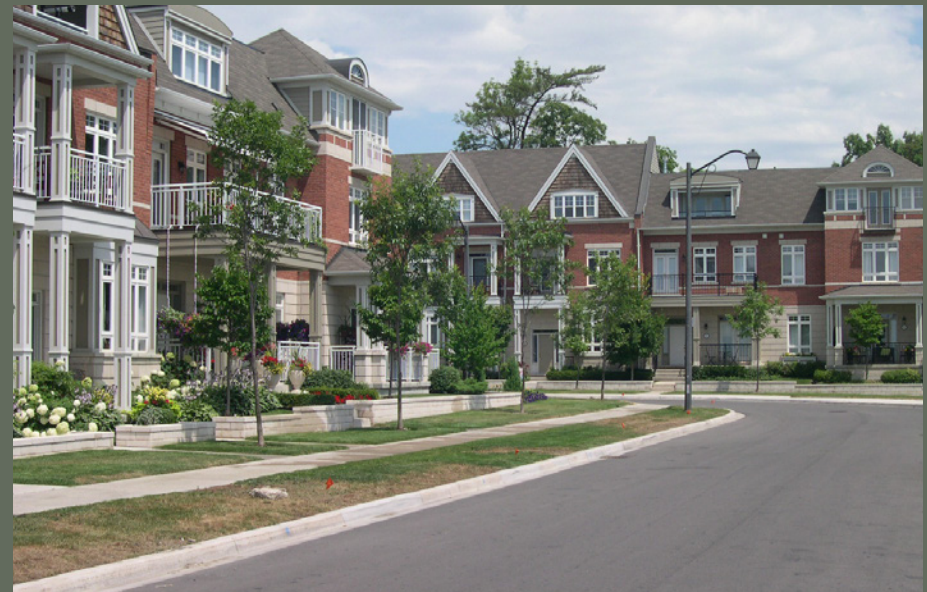
Image example of a towns with enhanced front elevations at a view terminus location.
