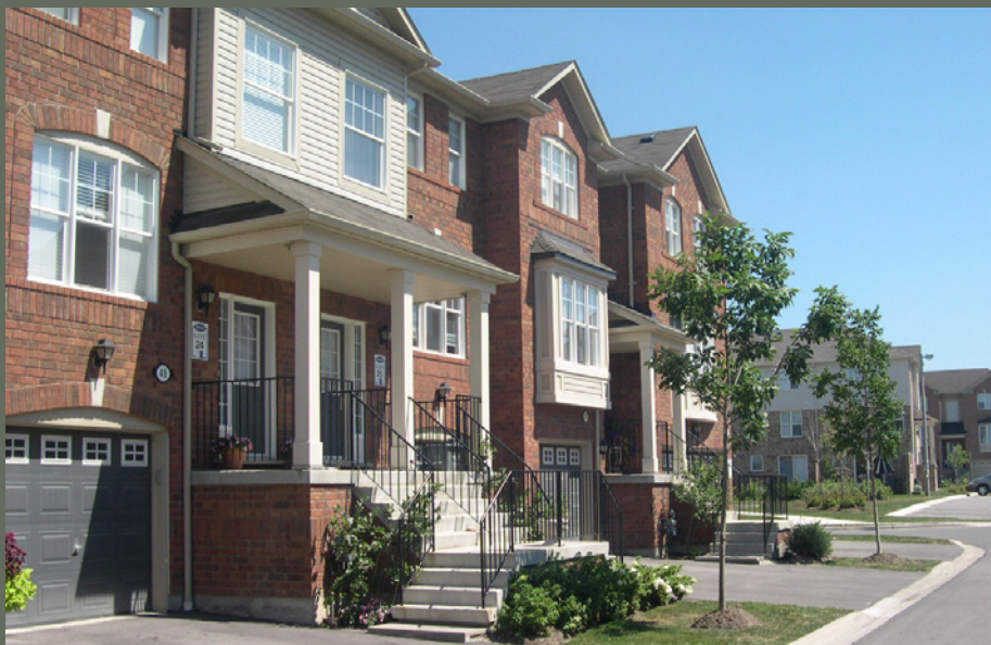
Image example of front-loaded townhouse units with garages integrated into the main building massing.
