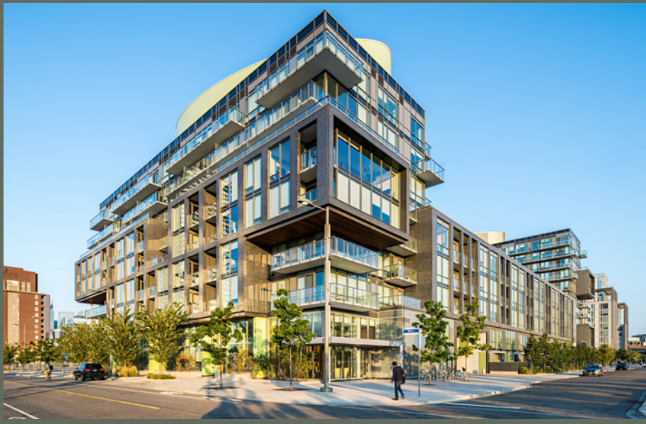
Image example of building height and massing that is concentrated at the corner location to ensure proper transitions to adjacent surroundings.
