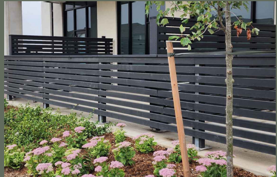
Image example of a wood slat privacy fence for ground units that will contribute to the building treatment at-grade/street interface.
