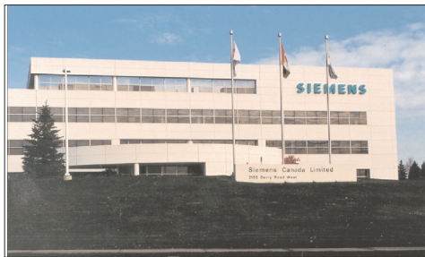
Photo 22 Buildings at Primary Gateways should be prominent and of high quality.
