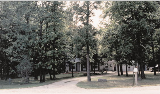
Photo 15 Esquesing Line existing residential use within mature landscape setting.
