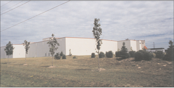
Photo 2 Long unarticulated street facades.
