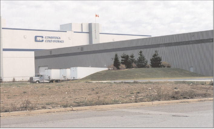
Photo 24 Screen loading areas from public view.
