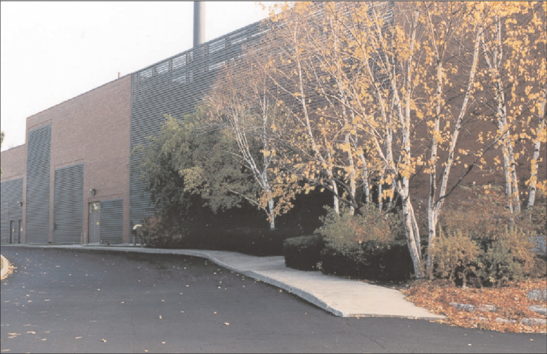
Photo 27 Screen mechanical penthouses as integrated building elements.
