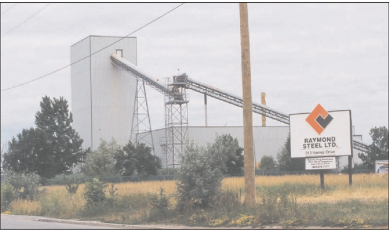
Photo 6 Existing heavy industrial uses.
