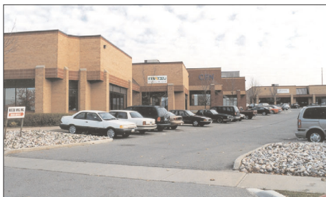
Photo 23 Articulation of the building elevation improves exposure for individual businesses.
