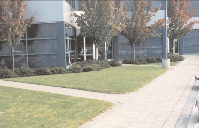
Photo 31 Walkways should provide direct pedestrian access from parking areas to main building entrances.
