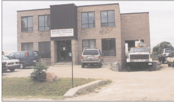
Photo 9 Industrial use with loading area facing the street.
