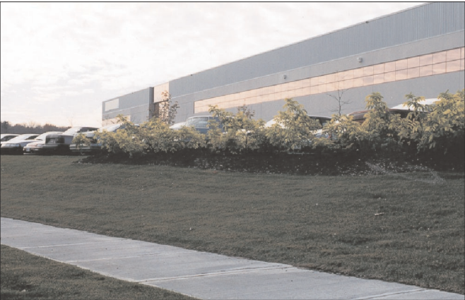
Photo 30 A 1.2 metre maximum screen height allows views into parking areas from the street, enhancing public safety.
